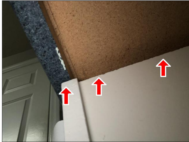
4.4 Item 2(Picture) Mud Room Counter Top
