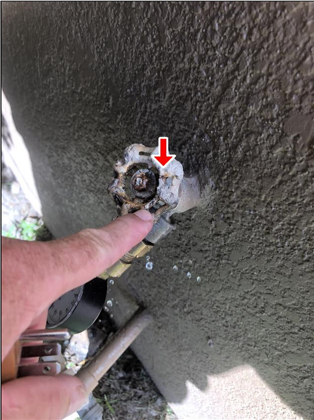
6.1 Item 1(Picture) South Side
