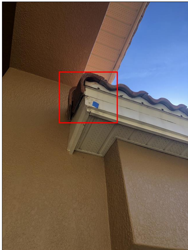
2.5 Item 6(Picture) West Side
