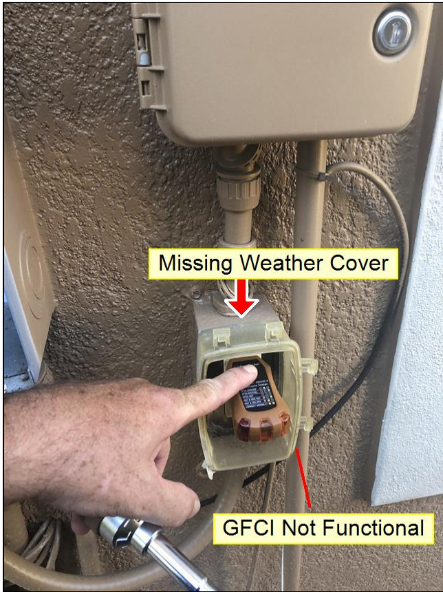
7.5 Item 1(Picture) North Side Exterior
