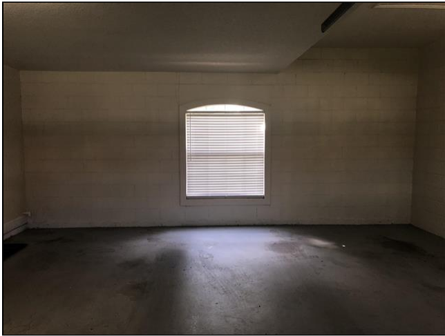
3.1 Item 3(Picture) South Wall
