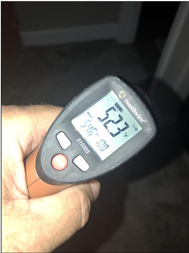
8.8 Item 9(Picture) Supply Air Cooling Temp
