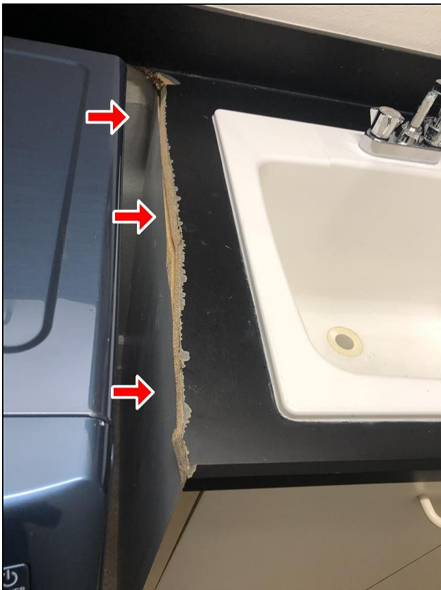
4.4 Item 3(Picture) Laundry Room
