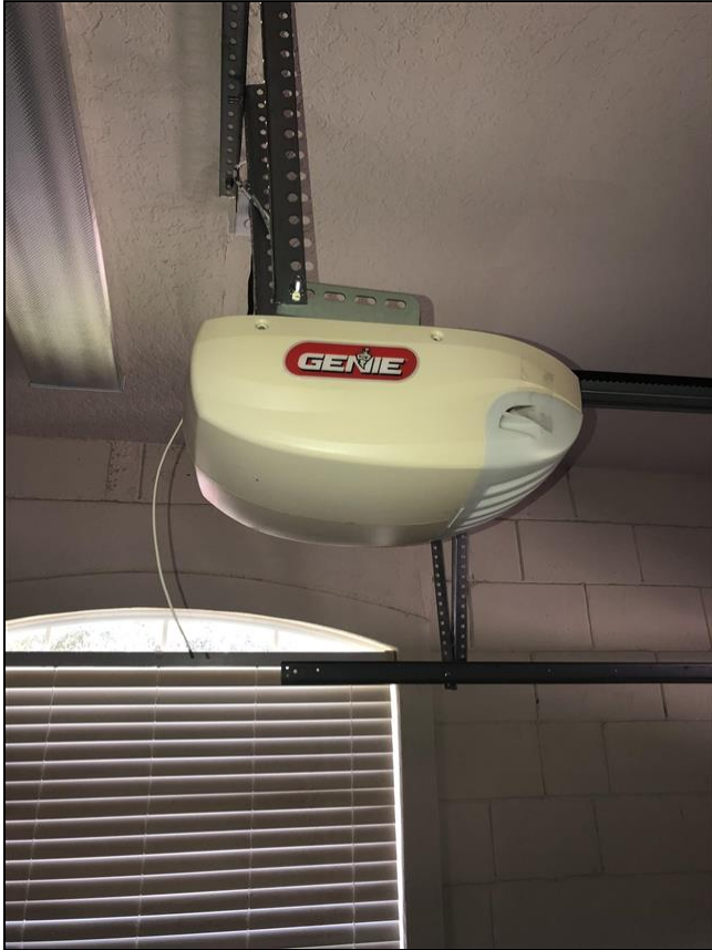
3.5 Item 1(Picture) Single Car Garage Door Operator
