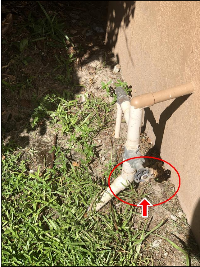
6.3 Item 1(Picture) South Side
