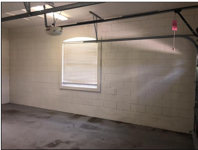
3.1 Item 1(Picture) West Wall
