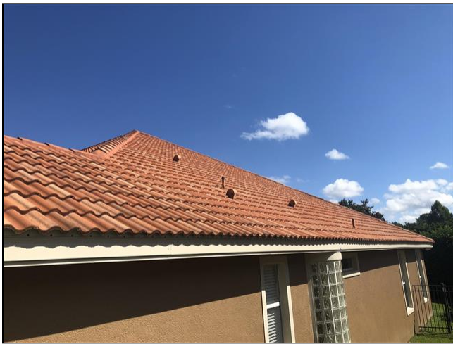
1.0 Item 1(Picture) Roof View
