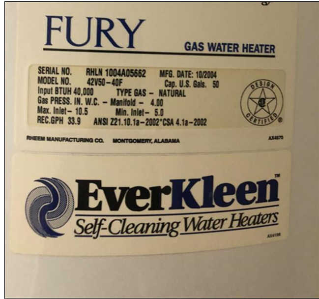
6.2 Item 4(Picture) Hot Water Heater Label
