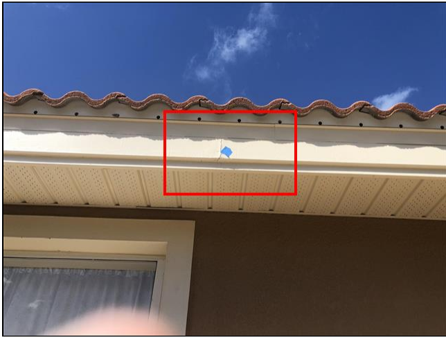
2.5 Item 3(Picture) South Side
