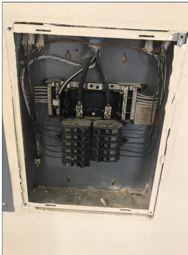
7.6 Item 8(Picture) Sub Electrical Panel B With Cover Removed
