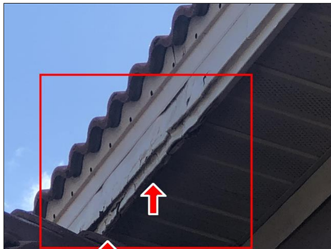
2.5 Item 2(Picture) North Side
