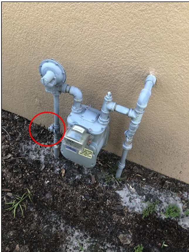
6.5 Item 1(Picture) North Side
