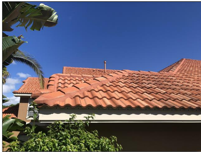
1.0 Item 2(Picture) Roof View
