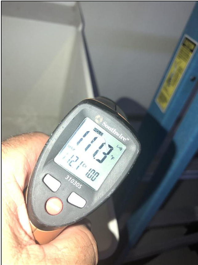
6.2 Item 1(Picture) Hot Water Temp
