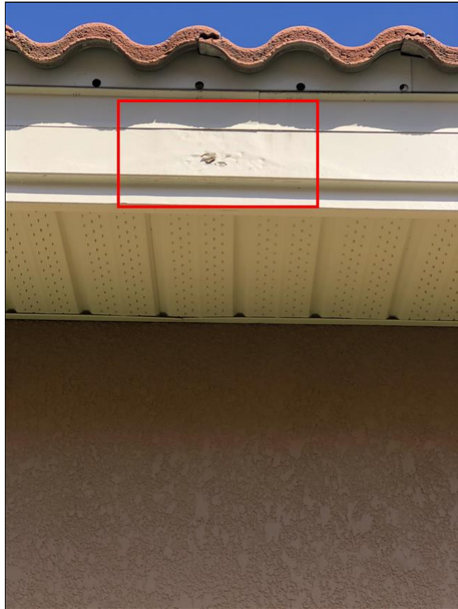
2.5 Item 4(Picture) South Side
