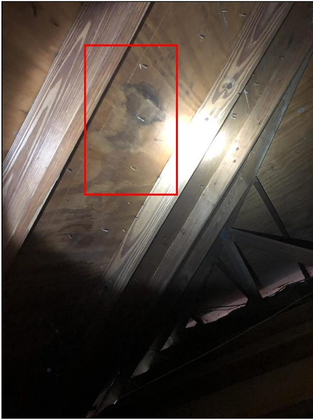
3.0 Item 3(Picture) Attic View Above Garage .
