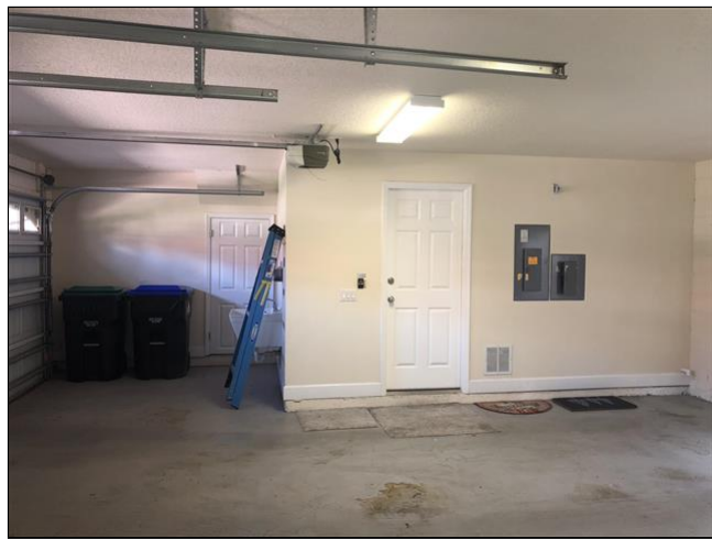
3.1 Item 2(Picture) East Wall
