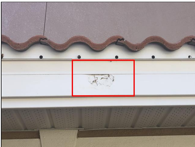
2.5 Item 1(Picture) North Side
